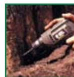
2. Drill a series of small 1" deep holes around the tree at the root flares.
